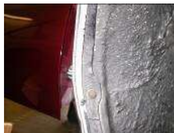
BOLTS AROUND WHEEL OPENING.
