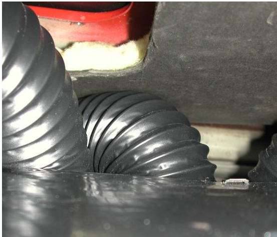
VIEW LOOKING UP THE REAR OF EVAPORATOR
