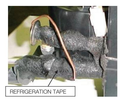
Locate in the hardware sack kit the refrigeration insulation tape. Wrap all of the exposed metal surface from the unit to the insulation on the tube.
